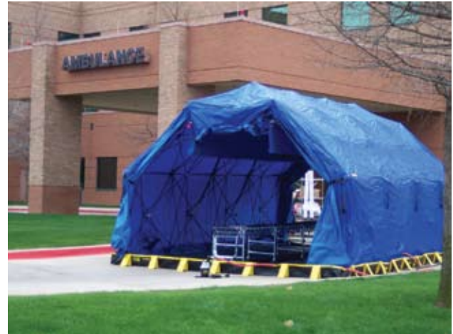
Fig. 16-6. A medium sized Reeves DRASH (deployable rapid assembly shelter). The scissors construction allows for tent expansion similar to the TVI tent but with the framework on the inside of the shelter. It also has integrated plumbing and a litter roller system. Can be configured for both ambulatory and litter patients. Photograph: Courtesy of Lt Col Charles Boardman, US Air Force, US Army Medical Research Institute of Chemical Defense. Reproduced with permission from Reeves EMS LLC, Orangeburg, NY.
